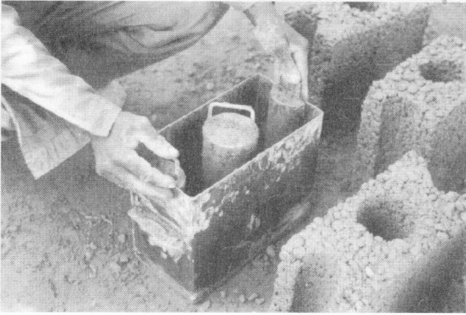
Placing internal moulds
