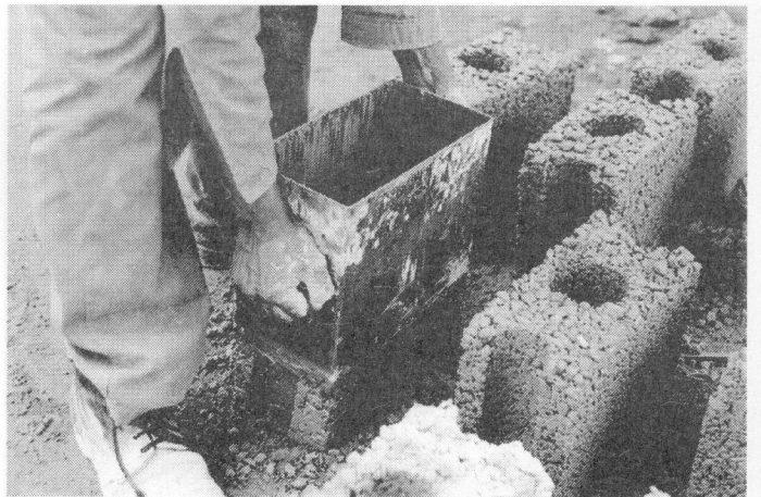
Lifting external mould
